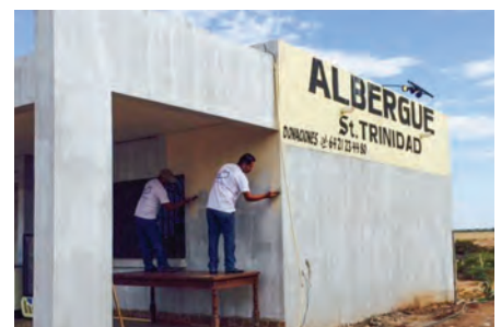
Maintenance work at the Holy Trinity Home
