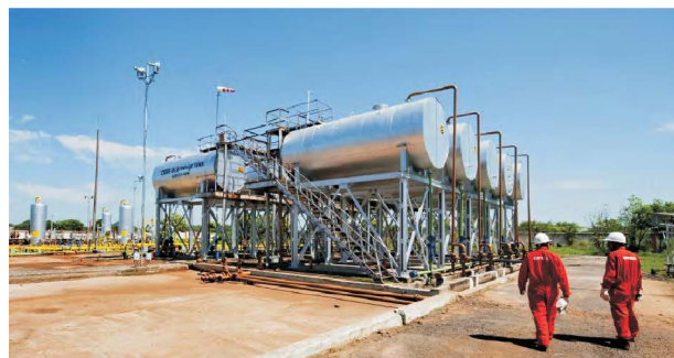
Crude oil storage tank in GGS, ONGC
