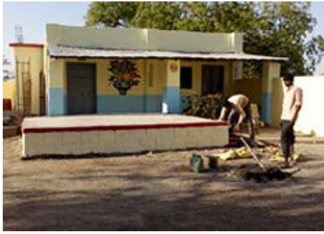
School Premise at Mohpuri Village
