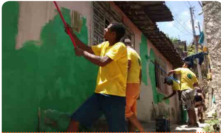
△ Employees in Brazil helped renovate buildings as part of TGVL.
