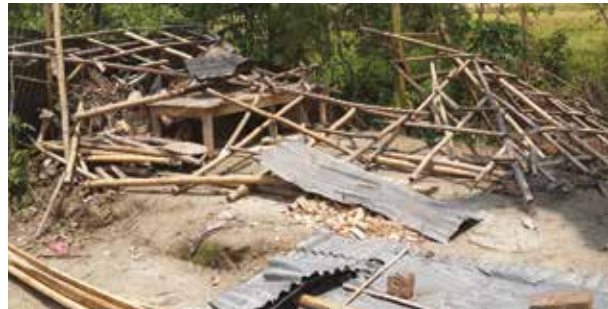
Catastrophe of the storm caused at Bogra
