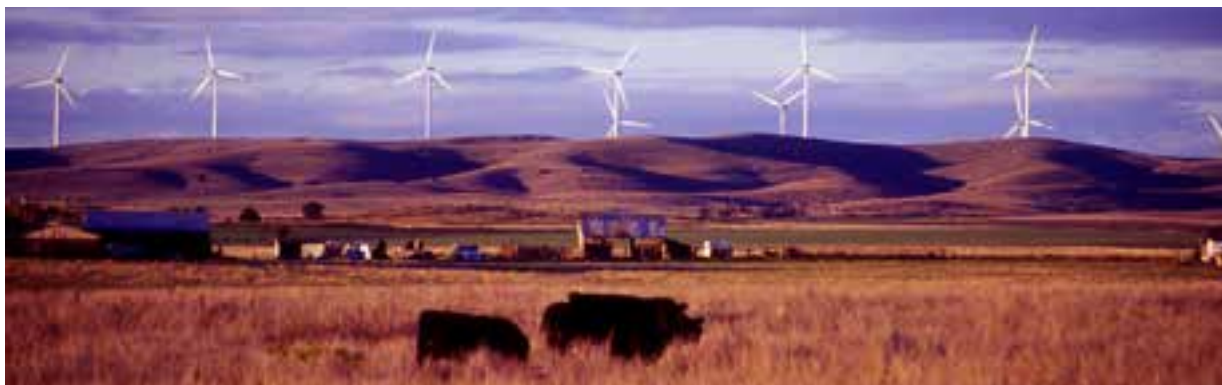
Blue Canyon Wind Farm, in USA
