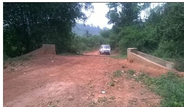
Plates 56 and 57: Show the culvert constructed at Pit A, near Akyem
