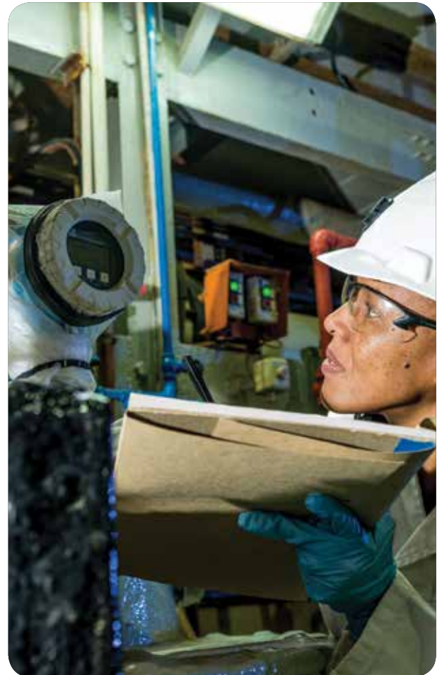
Inspecting a level indicator at one of the holding tanks at the PMR.
