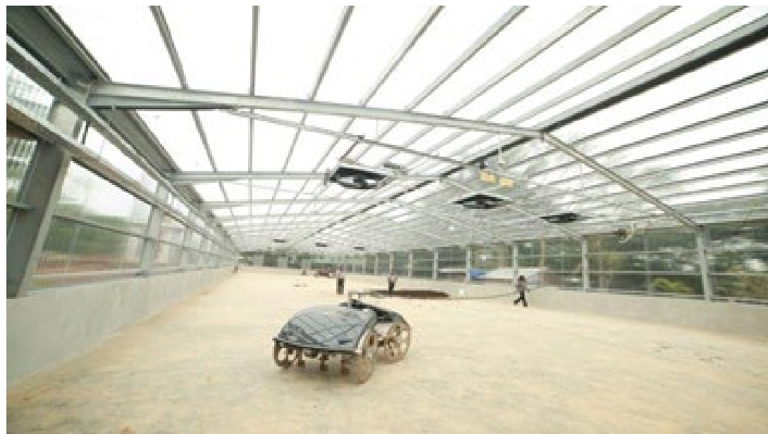
Built at a cost of USD 450,000 the 10,000 square foot sludge drying facility will help us to manage 1,600 tonnes of wet sludge per year by reducing it to 550 tonnes of dry sludge that will then be used as a co-processing fuel under strict controls.
