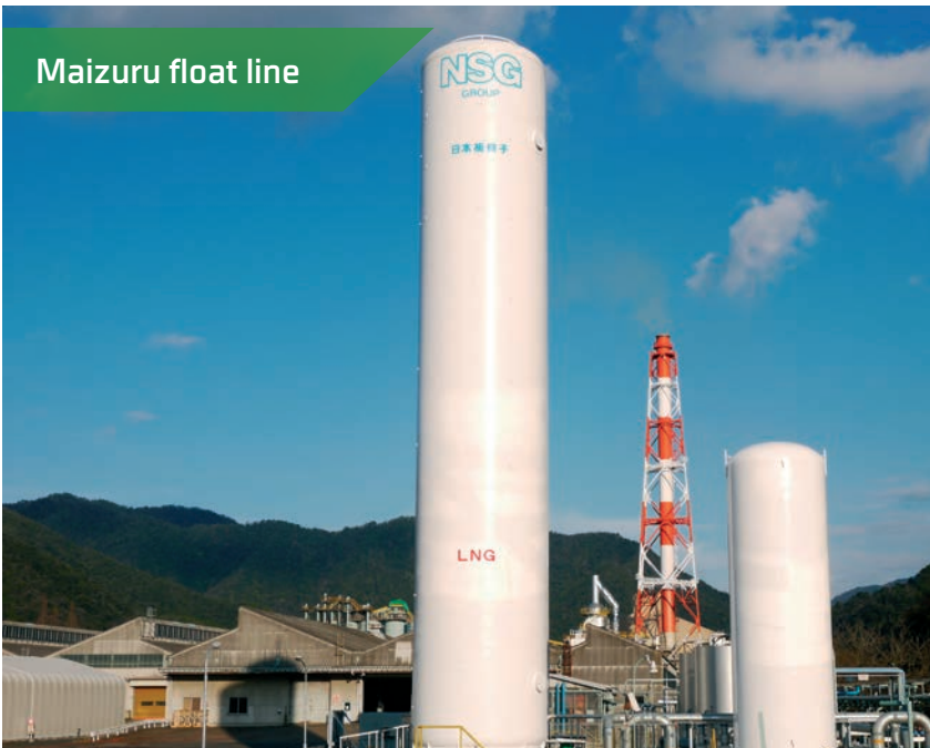
A large-scale project to shift the Maizuru float line M5F from heavy fuel oil to liquid natural gas stored in two large tanks reduced overall fuel costs and provided a significant reduction in CO 2 emissions. The reduced sulfur content also allowed simplification of the flue-gas desulfurization equipment.
