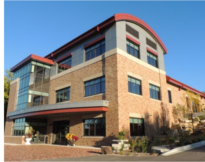
The da Vinci Center, which houses facilities and engineering, opened its doors in June of 2014.
