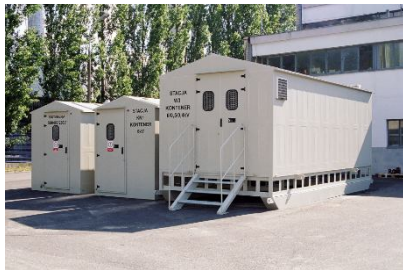
container transformer and distribution substations
