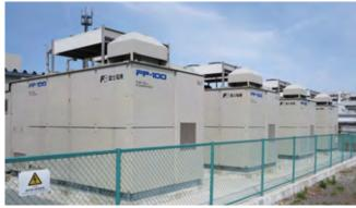
Fuel cells installed at a model factory (Yamanashi Factory) under Fuji Electric's Smart
