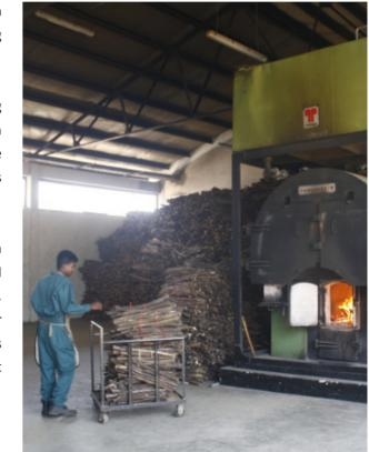
In addition it offers several other technical advantages such as high calorific value (4900 kcal/kg) and density compared to other commonly used wood such as rubber, low ash content (0.86% by weight) and less smoke generation than other wood based fuel. It also serves to benefit the community as Cinnamon wood is purchased from local suppliers and provides an additional income to the farmers and the local supply chain.
