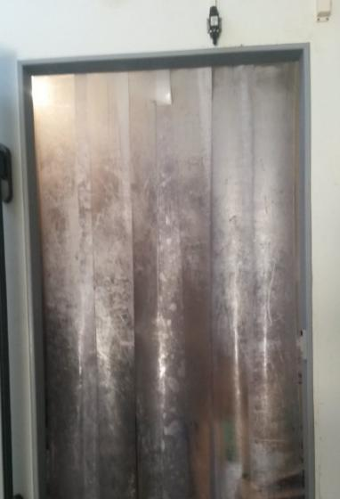
Energy loss through cold rooms has been reduced through the installation of freezer curtains and carefully monitored door opening schedules.
