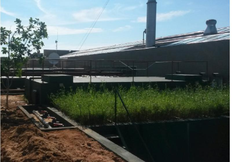
Prewash and main wash water and final rinsing water from the laundry is collected and treated separately. The treated final rinse water is used as primary wash water in the laundry. By doing so, fresh water consumption is reduced by 30% in laundry processes.
