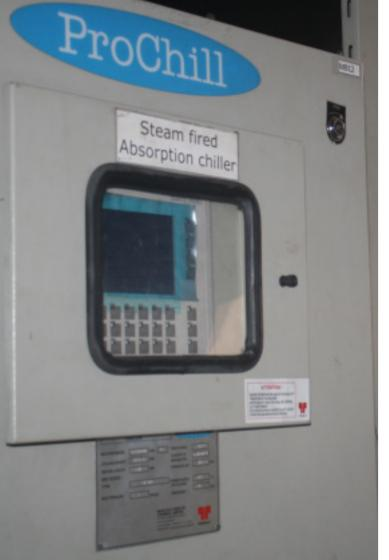
Since there are no high capacity compressors not only is the electrical power consumption very low, it produces less noise and requires less maintenance too. Since water is used as the refrigerant, unlike CFC/HCFC gas (which are ozone depleting substances) it is environment friendly — with no air pollution during repairs or if there are any leakages - and there is no recurring costs for refrigerants.
