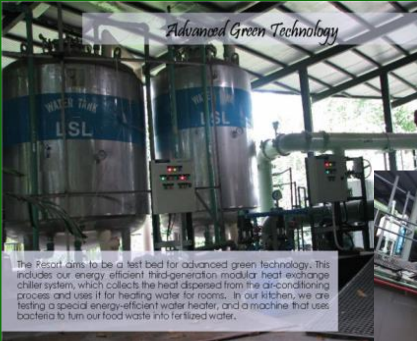
4 th generation modular heat exchange chiller system.
