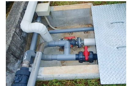
Status of work to uncover buried pipes (Kochi Factory)
