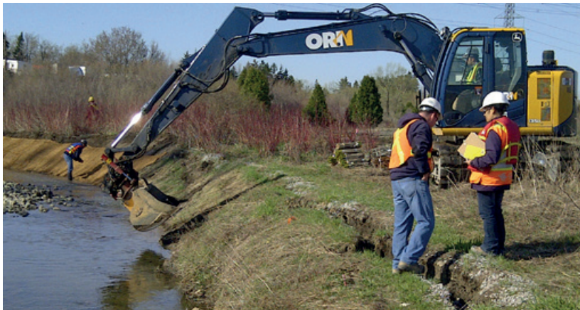
Stabilization of the banks of Black Creek along the area of influence of the construction work.
