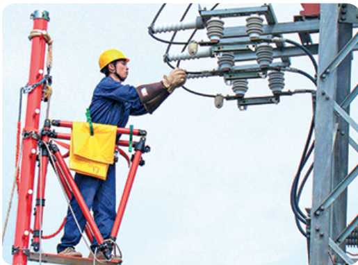
Insulated single foot ladder independently developed by Guangzhou Power Supply Bureau, giving more freedom to on-load operations
