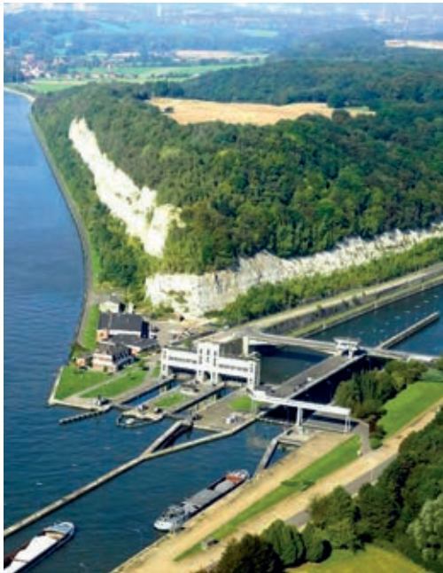
BELGIUM – LANAYE LOCK FACILITY: all work on electromechanical systems for the Lanaye waterway lock project, comprising renovation of three locks and construction of a fourth.
