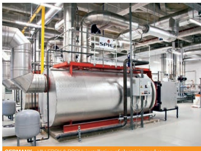
GERMANY – VILLEROY & BOCH: installation of electricity and steam cogeneration unit bringing energy savings of around 25% and reducing CO 2 emissions by more than 5,000 tonnes per year.
