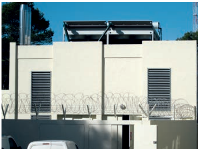
FRANCE – TDF: installation of very-high-energy-efficiency data centre, with two mechanical-compression-free cooling units.
