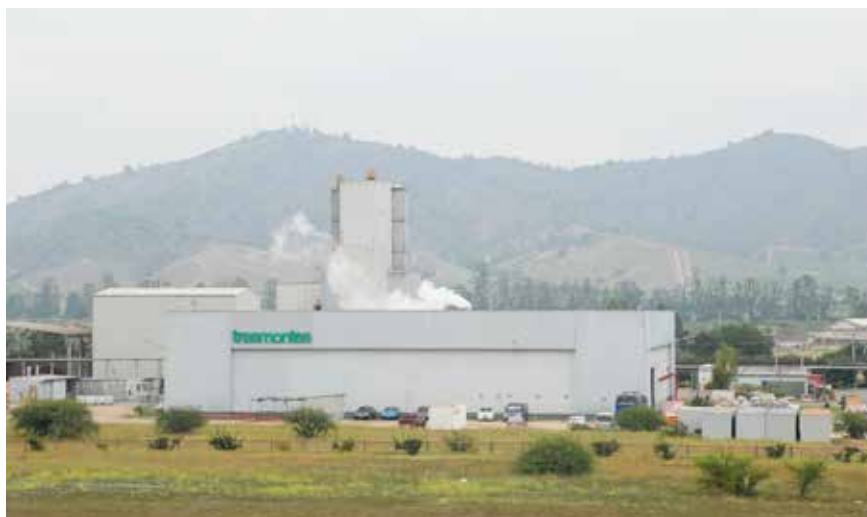
Tresmontes Lucchetti Business Industrial Complex in Casablanca, Chile.
