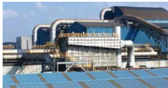
Dust collector installation at Pohang Works
