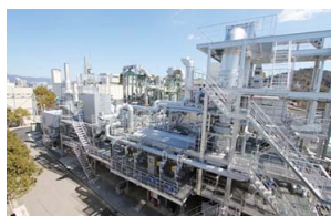
Sludge-Fueled Power System Demonstration Plant Treatment capacity: 35 wet tons/day (with moisture content of about 70%) Generating capacity: About 100 kWh/h
