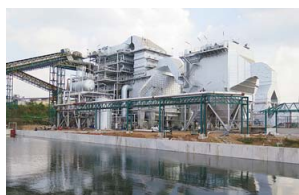
Bagasse Fired Boiler Plant (Thailand) Capacity: 165 tons/hour ×10.5MPa×520°C
