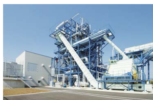
Wood Chip Biomass Power Plant (Kochi Prefecture) Generating output: 6,250 kW
