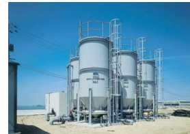
Continuous up-flow sand filter
