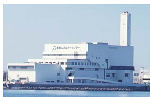
Wakayama Aogishi Energy Center Primary equipment improvement project Treatment capacity: 400 tons/day Generating output: 4,300 kW
