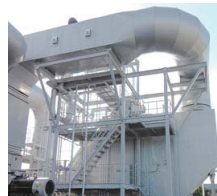
Waste heat boiler
