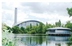
Energy from Waste Plant (UK) Treatment capacity: 1,370 tons/day Generating output: 36,650 kW
