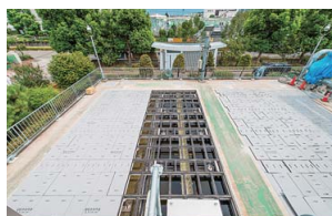
Osaka Hirano Sewage Treatment Plant Upflow moving bed sand filtration system (high-speed) Treatment capacity: 120,000 m 3 /day
