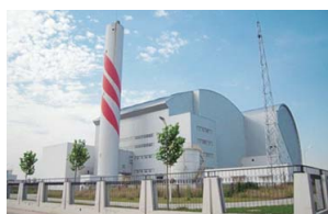
Energy from Waste Plant (Beijing, China) Treatment capacity: 1,600 tons/day Generating output: 30,000 kW
