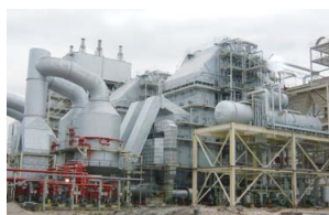
Bagasse Fired Boiler Plant (Thailand) Capacity: 125 tons/hour ×4.2MPa×485°C
