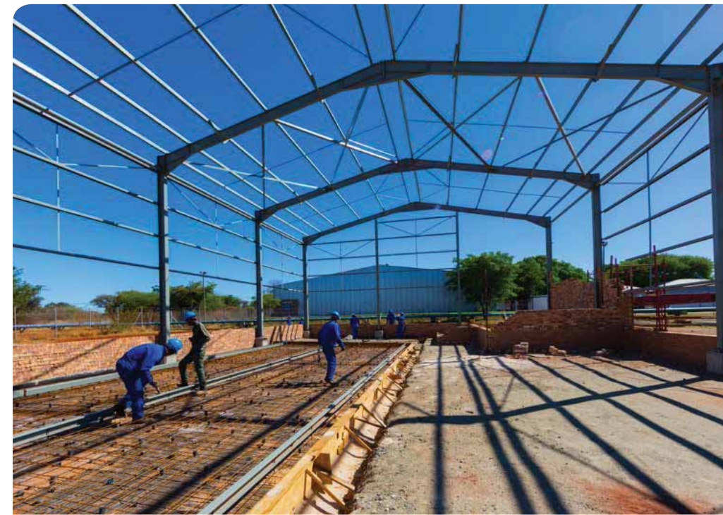
Phase I of the water treatment plant at BRPM under construction
