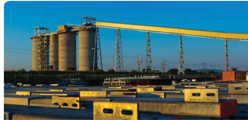
Styldrift I surface silos and feed conveyor
