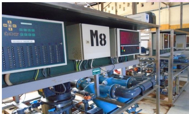
Newly installed computerized irrigation system
