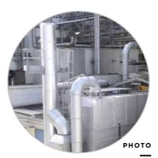
Regenerative thermal oxidation is used to reduce odor emissions by up to 99%.
