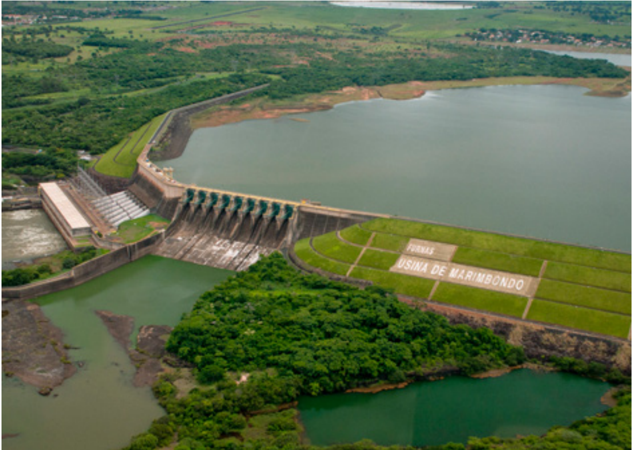
HPP MARIMBONDO (MG/SP)
