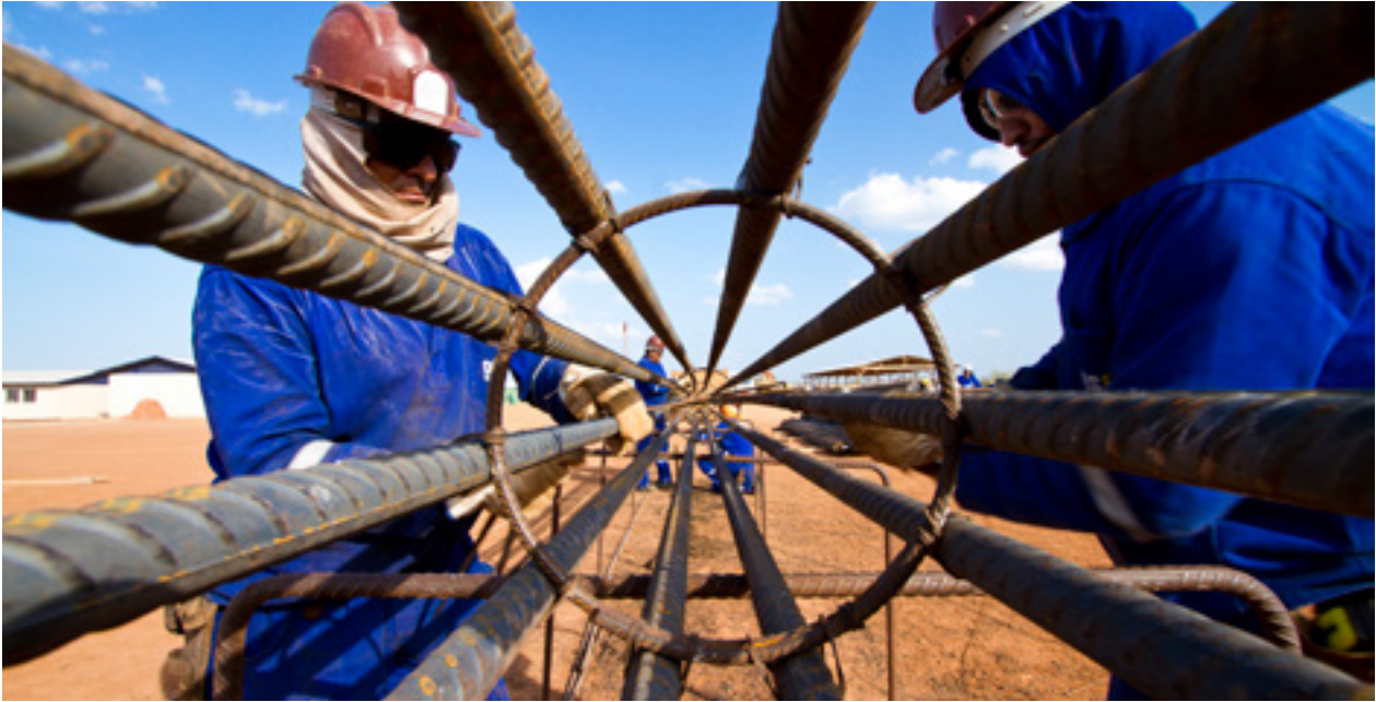
CONSTRUCTION OF THE MIASSABA III WIND FARM (RN)
