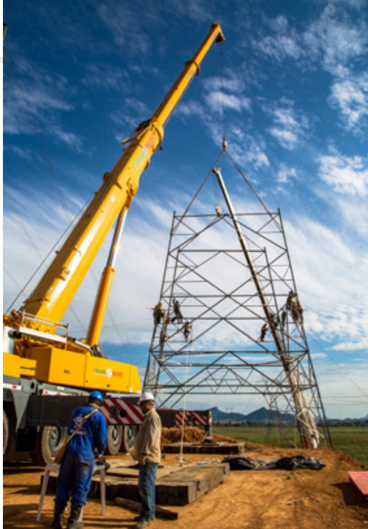
RECOVERY OF TRANSMISSION TOWERS/TL MACAÉ-CAMPOS (RJ)
