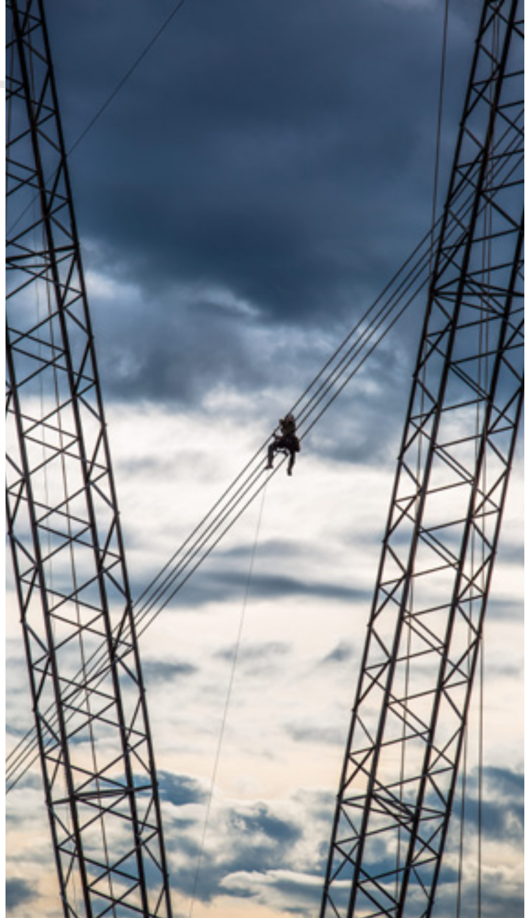
REPAIRING TRANSMISSION TOWERS - TL FOZ DO IGUAÇU-IVAIPORÃ (PR)
