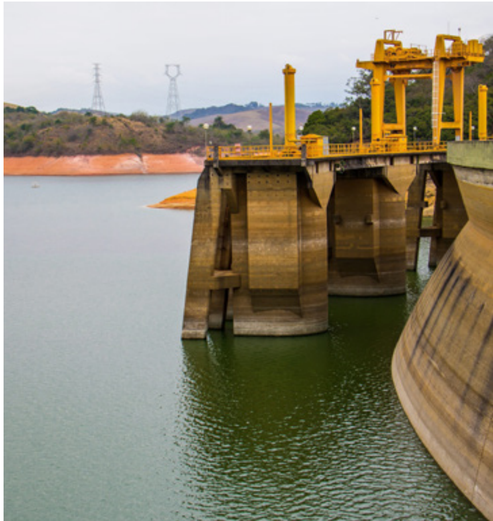
RESERVOIR AT HPP FUNIL (RJ)
