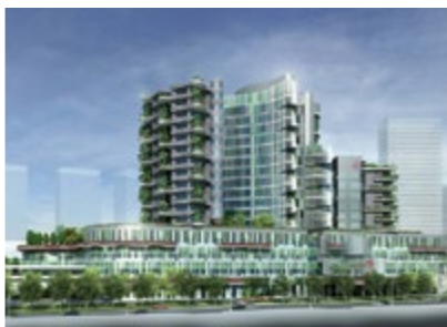
Ng Teng Fong Hospital • Location : Singapore • Project Period : 2012.06-2015.05
