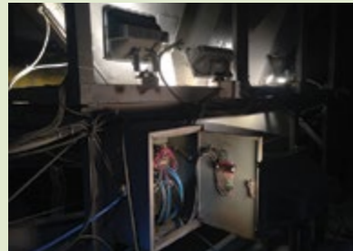
7th site for railroad construction in Wonju-Kangreung : Energy Saving and Net Zeroing of construction waste materials by utilizing halogen lights and freeze protection of equipments
