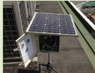
Down Town Line C937 Site : Energy-saving and reduction of noise complaint through operating the noise meter of solar energy generation
