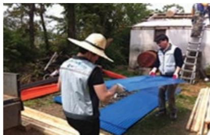
Total Number of House Repair of Hope 108 Houses
