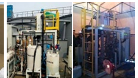
Metropolitan High Speed Railway(Suseo-Pyengtaek) Lot No.9 Project
