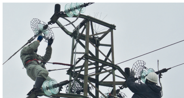
Colleagues from CSC Sliven install the new MST spacers. The photograph shows the already installed spiked protectors.
