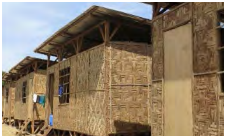
Above right: Philippines Transitional Shelter, 2011 Above: Philippines Transitional Shelter, 2012
