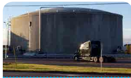
△ The waste water pre-treatment facility in Murfreesboro, Tennessee that removes dairy solids prior to discharging into the city treatment system.
