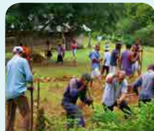
△ Pascal Hochedé from Arras helped dig the new school building foundation.
