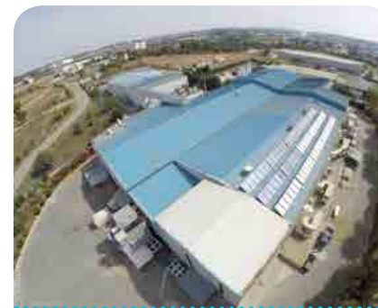
△ Solar panels at our facility in Inofita, Greece.
