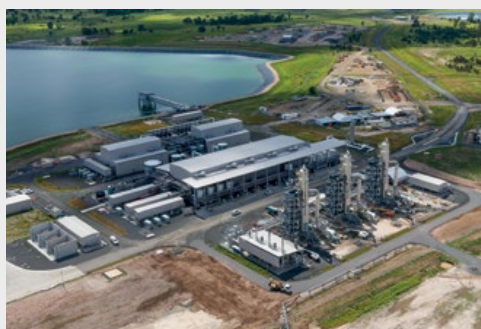
THE NORTHERN WATER TREATMENT PLANT
