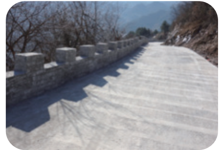
Village road reconstruction in An'hui
