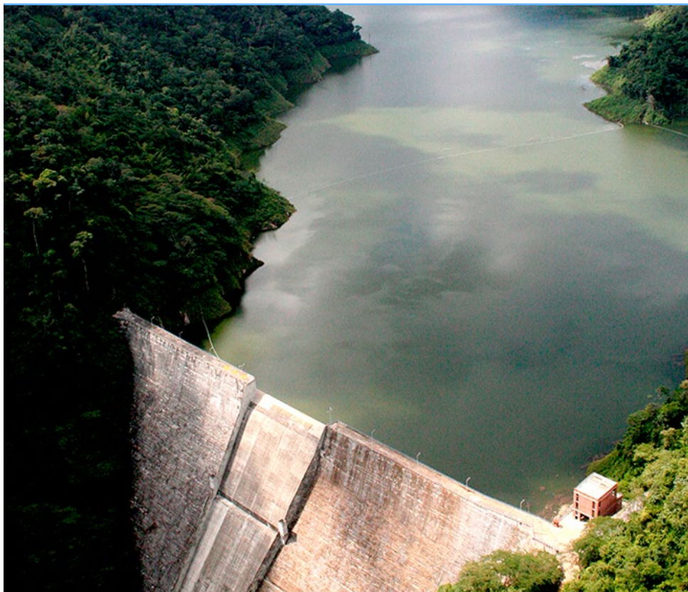
▼ Dam and Reservoir. Miel I Hydroelectric Power Plant.
