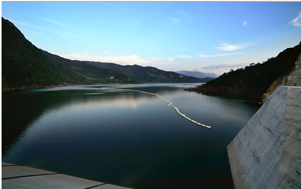
Topocoro Reservoir. Sogamoso Hydroelectric Power Plant.
