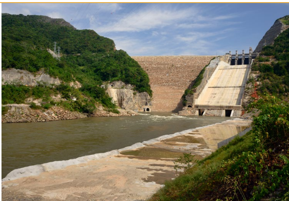
▼ Sogamoso Hydroelectric Power Plant.
