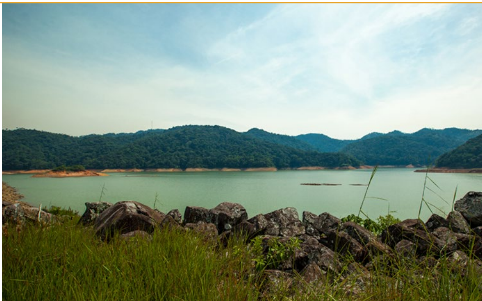
▼ Punchiná Reservoir. San Carlos Hydroelectric Power Plant.
