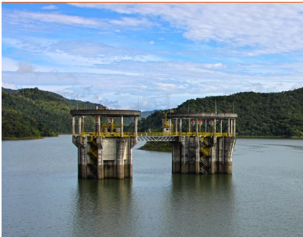
▼ Intake towers. San Carlos Hydroelectric Power Plant.
