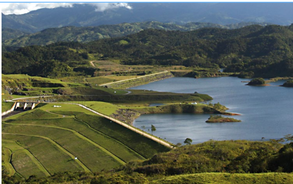
▶ San Lorenzo Reservoir. Jaguas Hydroelectric Power Plant.
