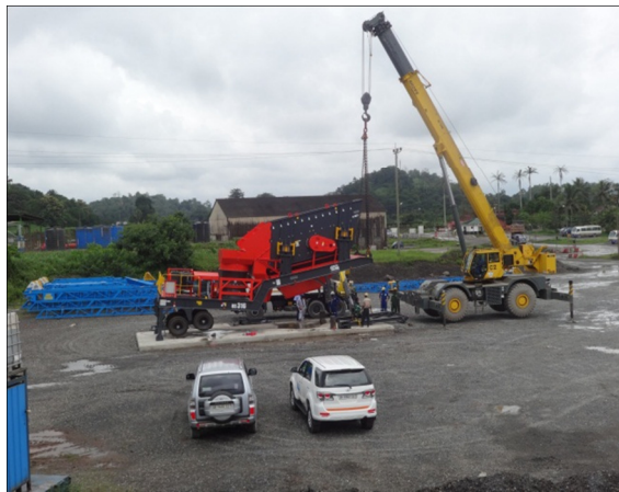
Plates 10 and 11: CPE – Foundation and installations – US 316 PLANT and US 316 Mobile unit with all conveyors connected
