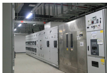
Low-voltage switch box
