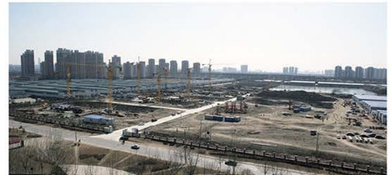
Shanty area renovation supported by Tianjin Branch
