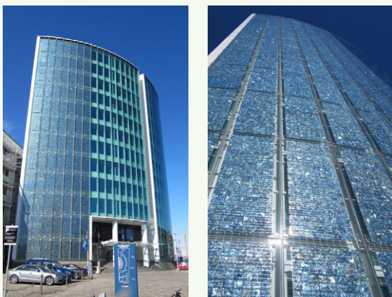
Pictured: ALM Brand building incorporating BIPV panels Pilkington Eclipse Advantage™ , Pilkington Optifloat™ , Pilkington Optiwhite™
