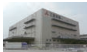
Tobishima Warehouse, Nagoya Branch
