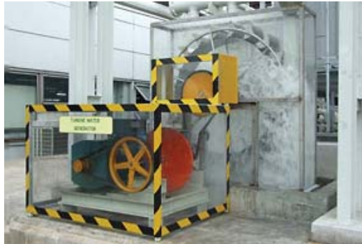
Hydropower utilizing cooling water from the plant
