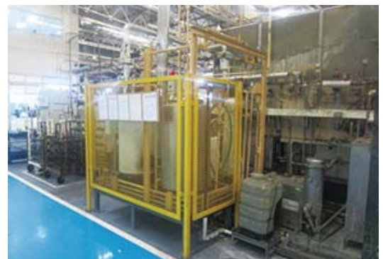
This boiler supply system was altered to reduce steam transmission losses (Daikin Compressor Industries Ltd.)
