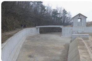
Repair of discharge channels and spillways
