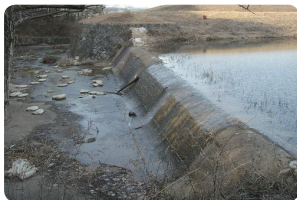
Obsolescence and damage of a spillway channel
