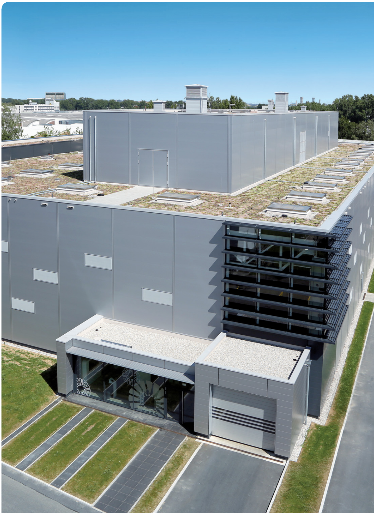
Sustainable construction: the new blisk production facility in Munich has a particularly energy-efficient design thanks to systematic heat recovery, cutting-edge ventilation technology and well-water cooling.
