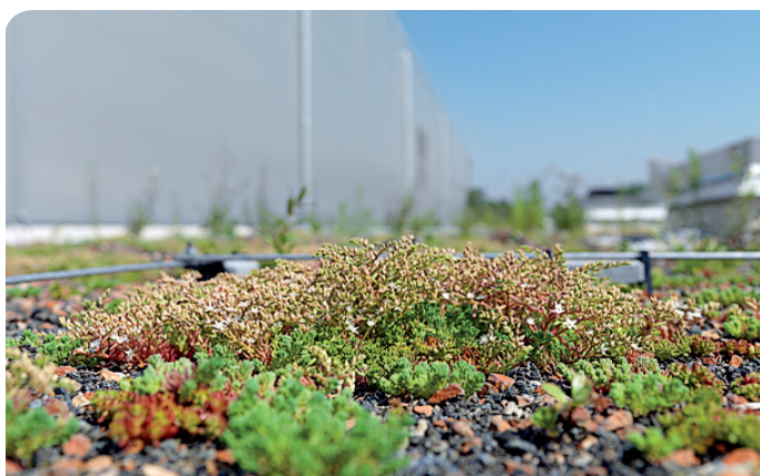
Green roofs: vegetation on top of buildings improves their insulation.
