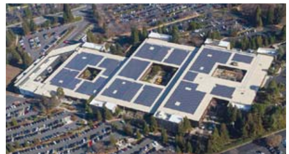
1 MW photovoltaic solar installation at HP headquarters, Palo Alto, California
