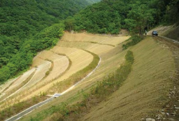
Completion of stabilization project of closed mine debris slopes
