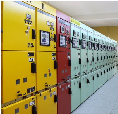
low and medium voltage switchgear
