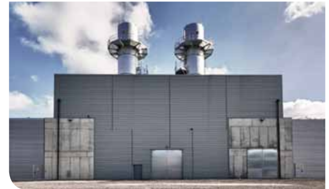
The fourth unit on the Angleur site, built in 2010, is an open cycle power plant with two 63 MW turbines that can reach full power in under ten minutes due to their low thermal mass. This “peak” power plant, as it is called, can supply the consumption peaks of 70,000 homes.
