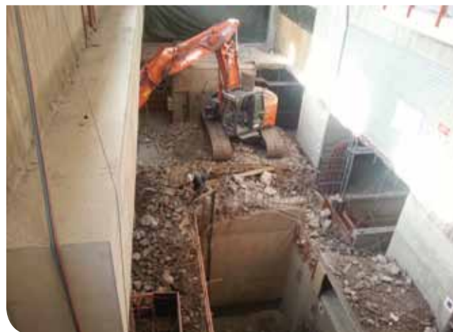
The demolition of part of the Lixhe hydroelectric power plant (here you can see the flues and the "engine room" level) generated a large amount of deconstruction waste, most of which was crushed and recycled.
