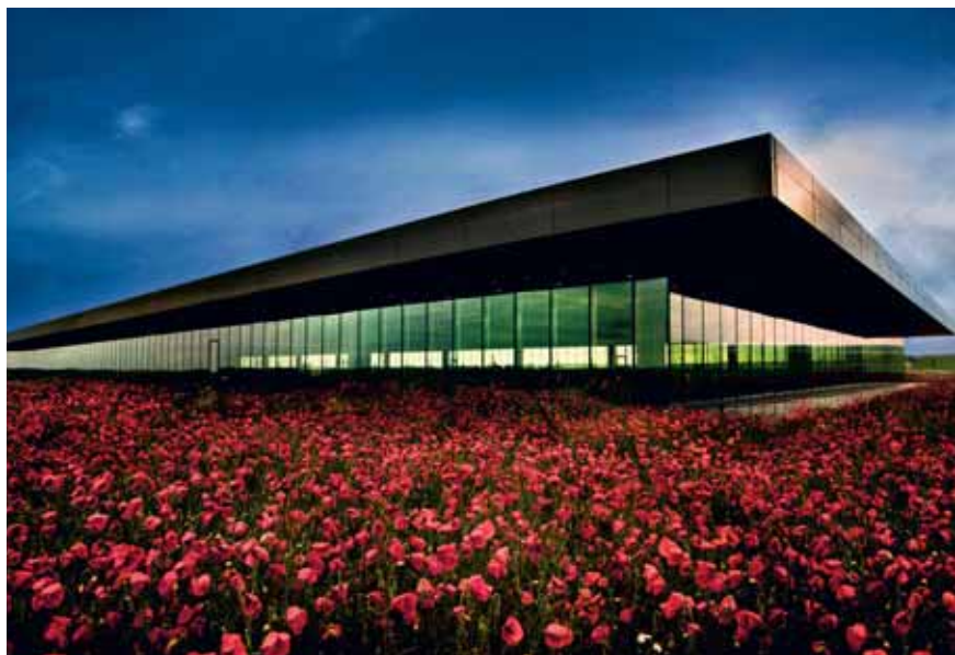
Moët & Chandon's HQE® fermenting room at Mont-Aigu.
