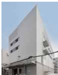
The Energy and Emergency Control Center
