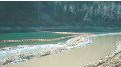
Installing Anti-Pollution Net
