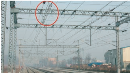
Catenary tensioning
