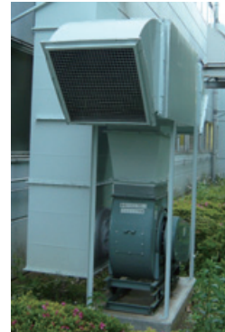
Exhaust vent with a noise reduction cover
