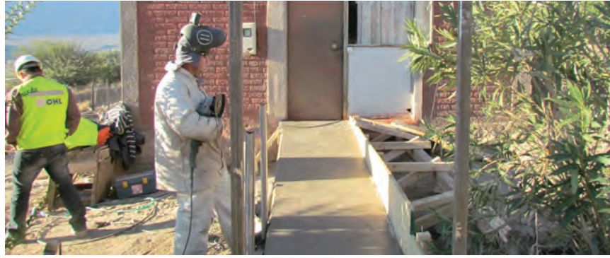
Construction of a wheelchair access ramp.
