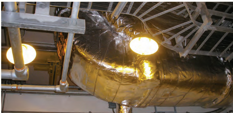
Protection installed with DUCT WRAP 100-3.
